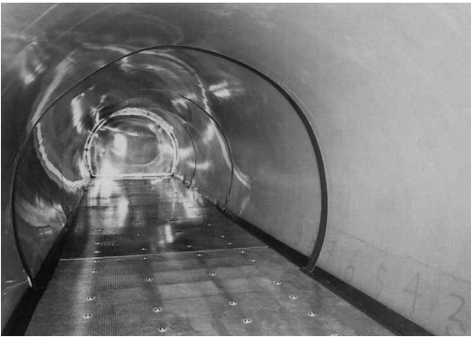
Fig. 6 Installation of the interior trim panel.
